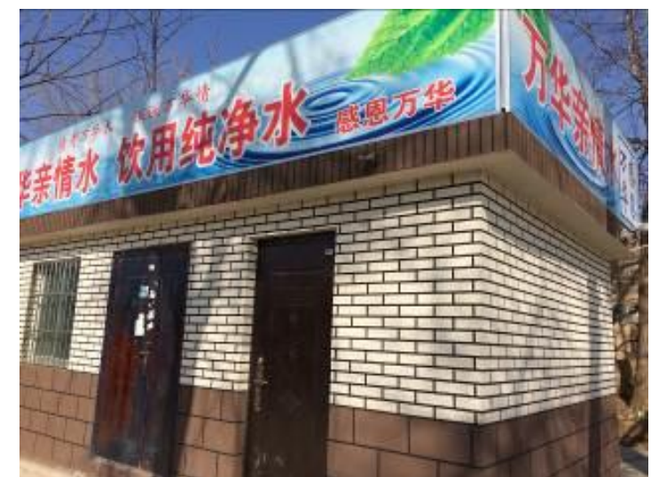
Wanhua treatment station of pure water
